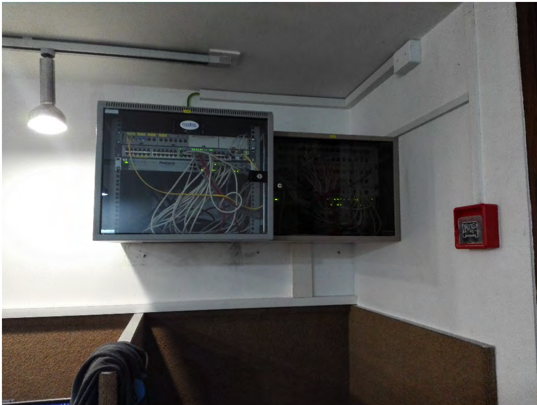
Figure 53: Original network installation – difficult to maintain
