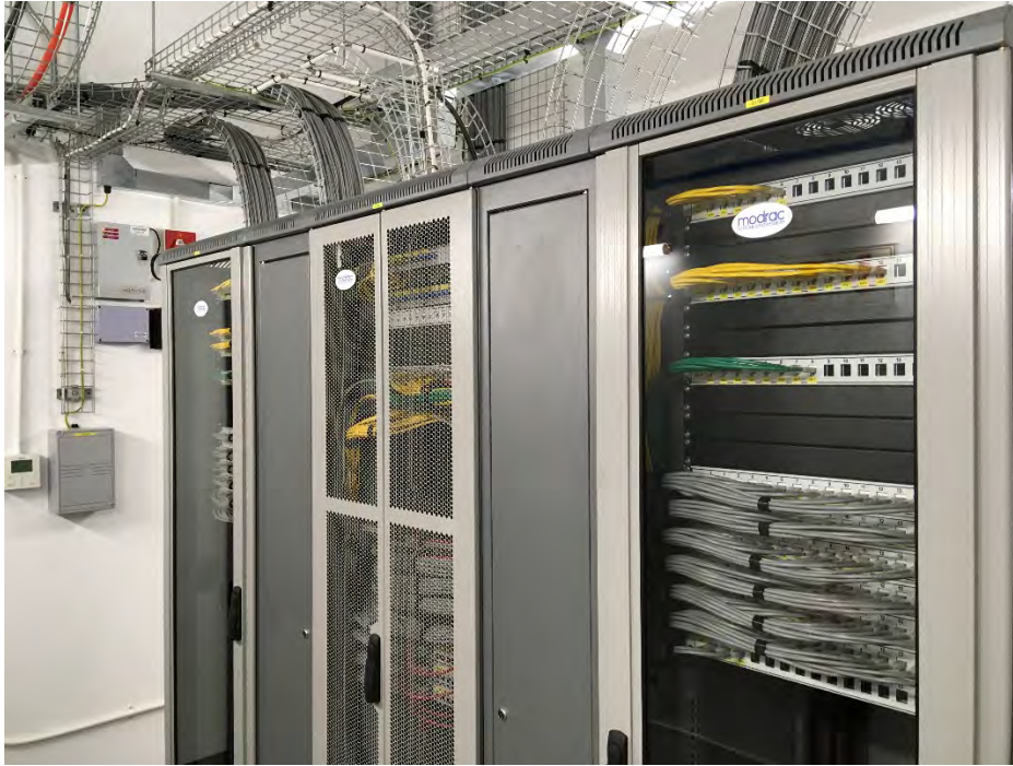
Figure 55: Large cabinets in central network distribution room for easier service access
