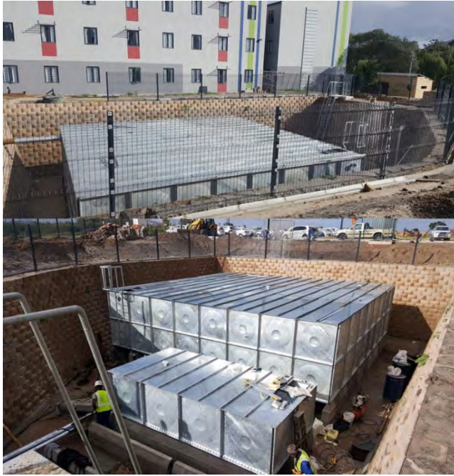
Figure 19: New 200 kl stormwater storage tank and 10 kl greywater storage tank being installed
